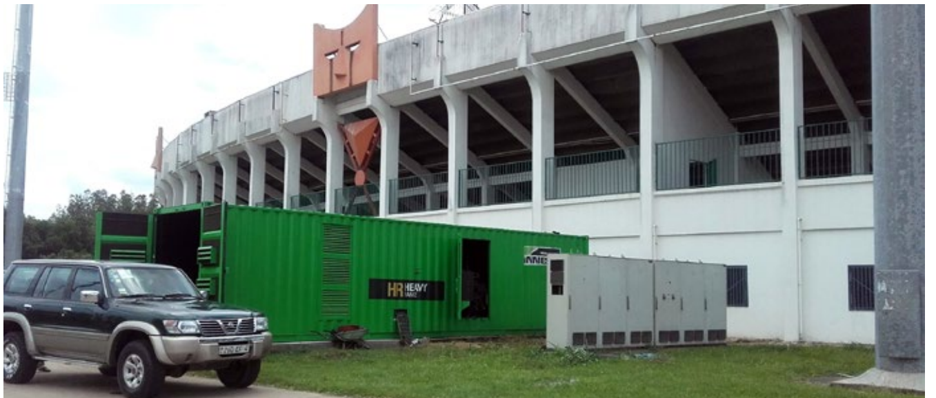
IP-1135 genset with dual soundproofing panel
