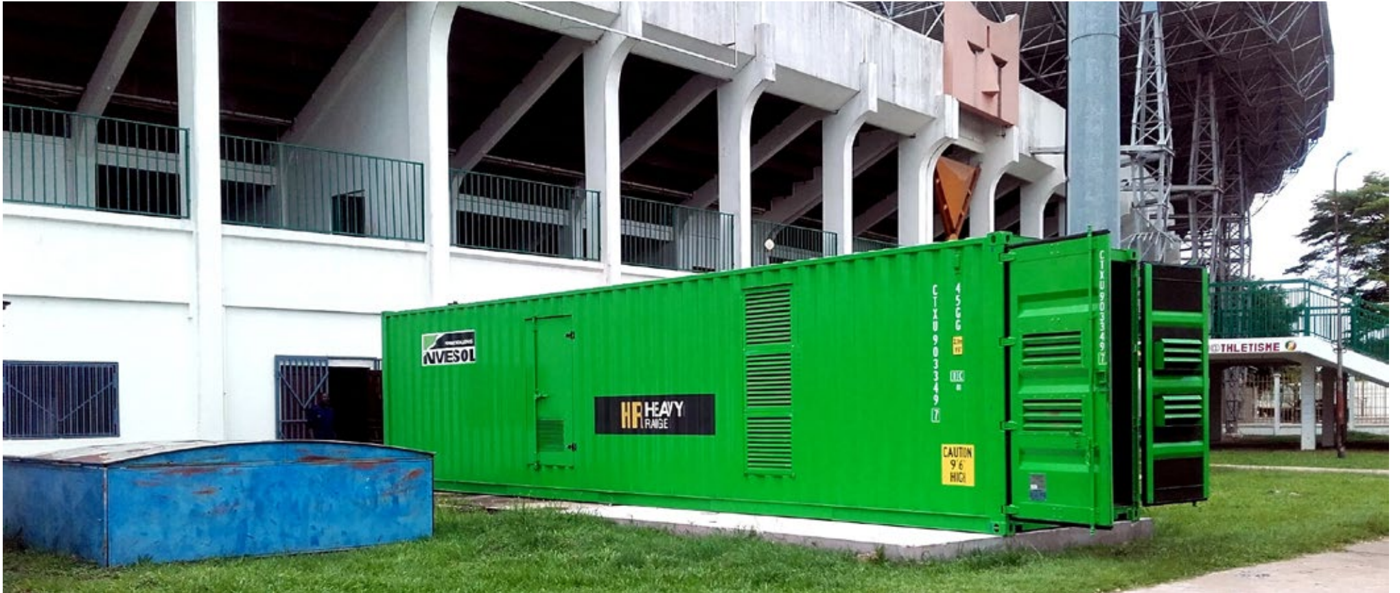
INMESOL stand-by generator set, model IP-1135
