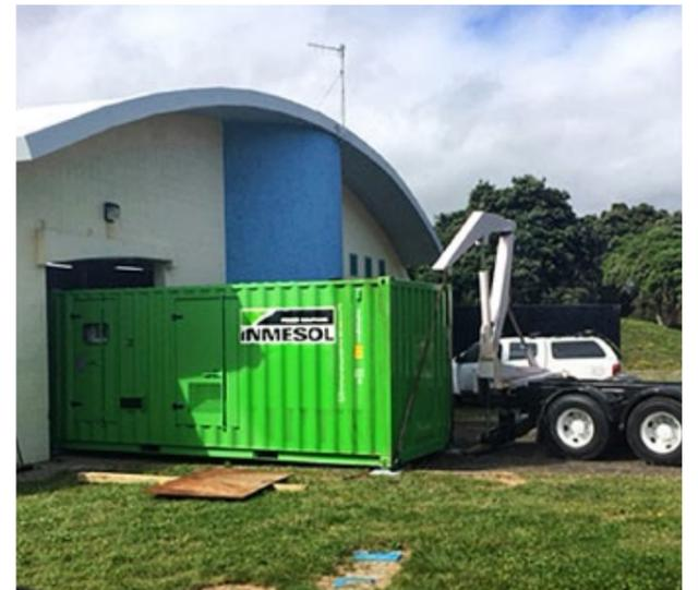
Genset model IT-1115 being placed at the pumping station facility
