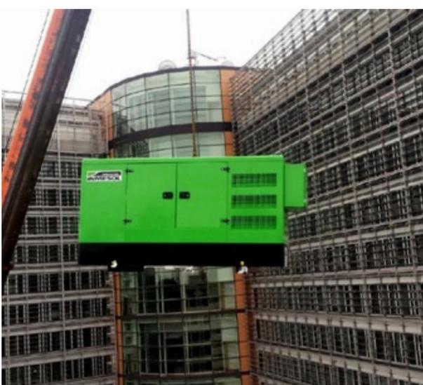
INMESOL stand-by generator set, model II-110, being lifted to the Berlaymont's roof
