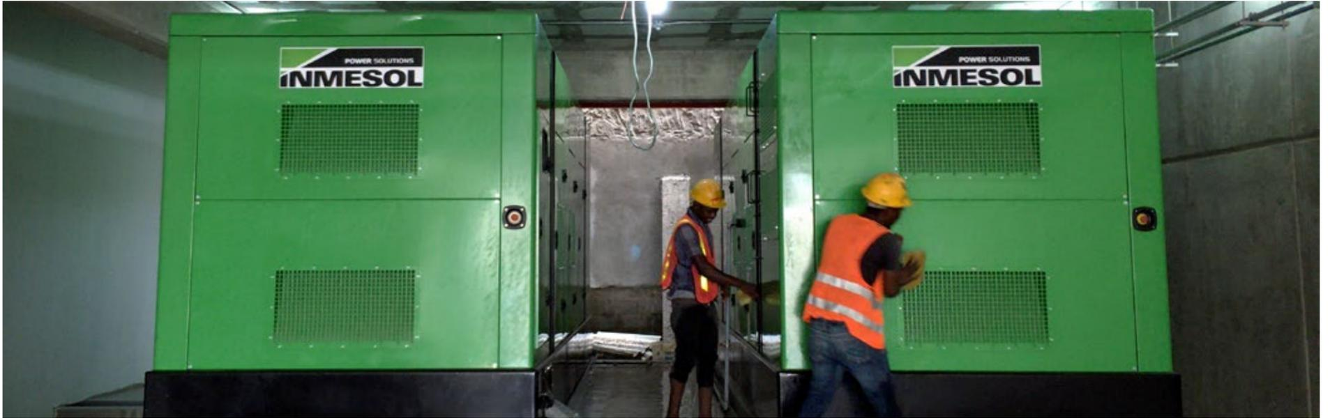
The two-genset 1010 kVA LTP power generation system recently installed in Las Colinas General Hospital basement
