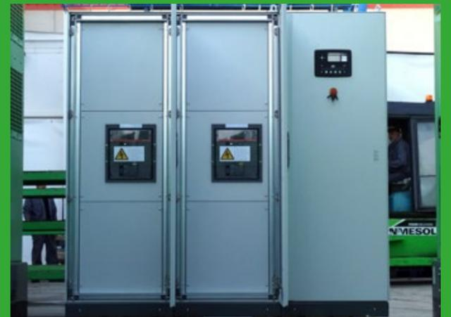
2500 A ATS panel, enabling the synchronised operation between both sets and the mains.
